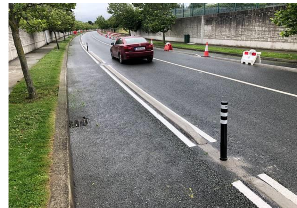
Figure 9: Retro-fit kerb solution (example shown is Benildus Avenue)
